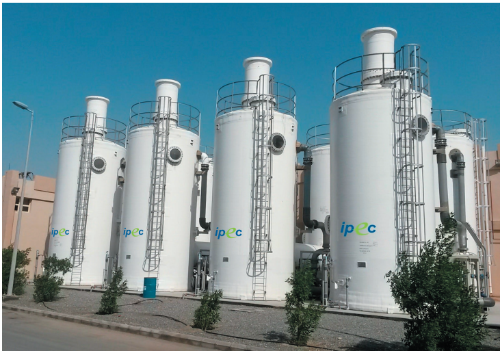
Jeddah South Pumping Station: 300.000m 3 /h two stage scrubber (Saudi-Arabia)
